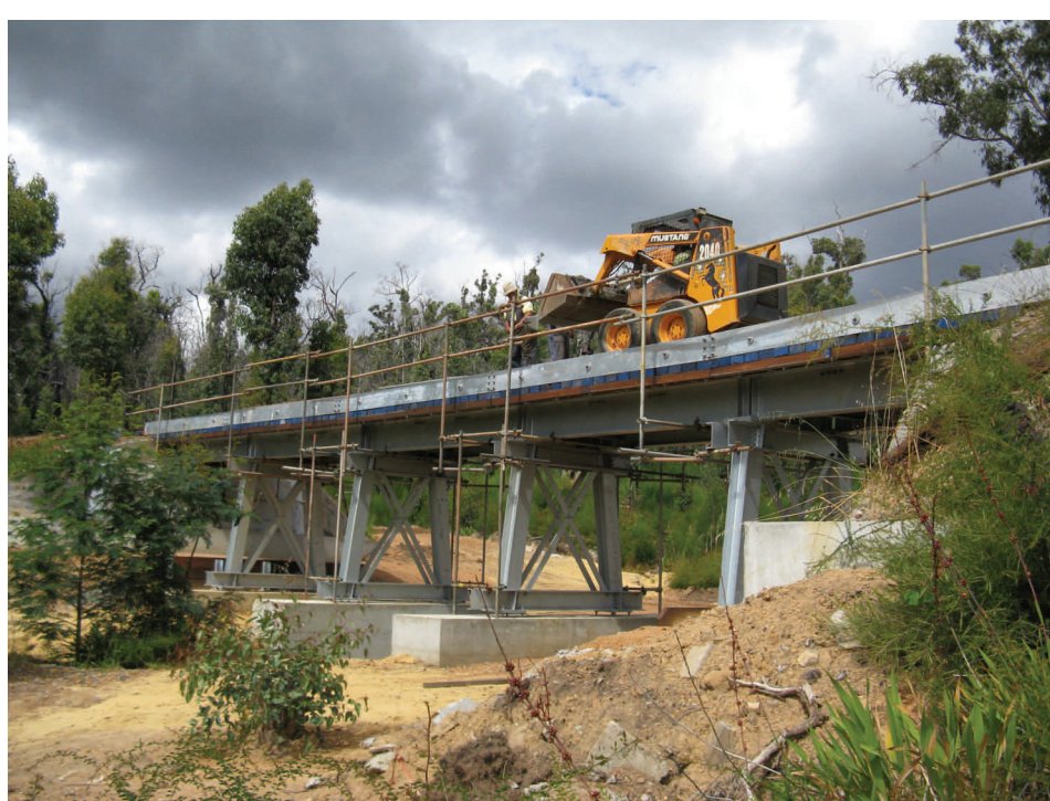
16km bridge – Restorative work by Hotham Valley Tourist Railway nears completion
