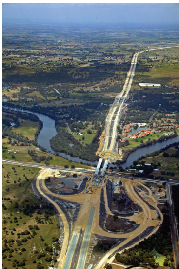
The Pinjarra Road Interchange and Murray River Bridge
