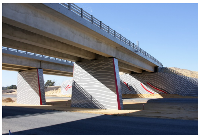
Mandjoogordap Drive Overpass
