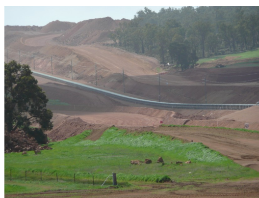
BHP Bauxite Conveyor System, Boddington (S)
