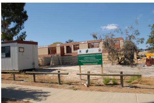
Boddington Medical Centre under Construction
